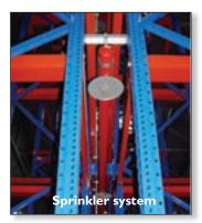
The sprinkler system is connected on the row spacers, which link the two frames of the double rack.
